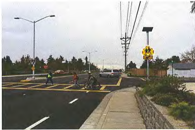
E Traffic Safety Improvement Project
