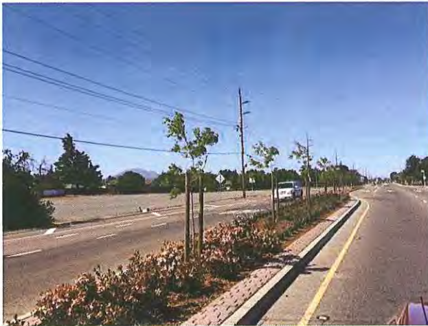
A Main Street Median Improvement Project
