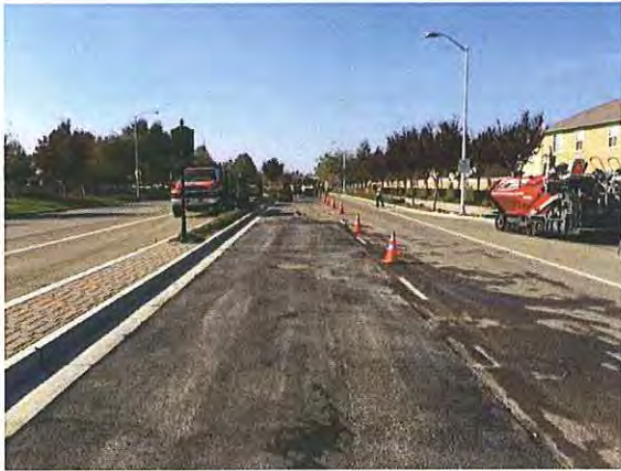
C Street Resurfacing and Repair Project
