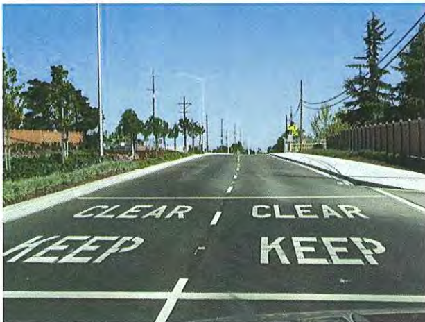
H City Street Restriping Project
