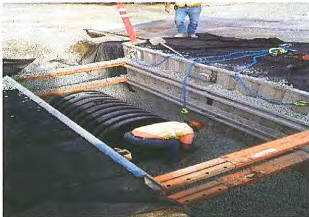
B Main Street Storm Drain Improvement Project
