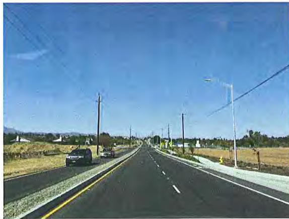
F Laurel Road Widening Project
