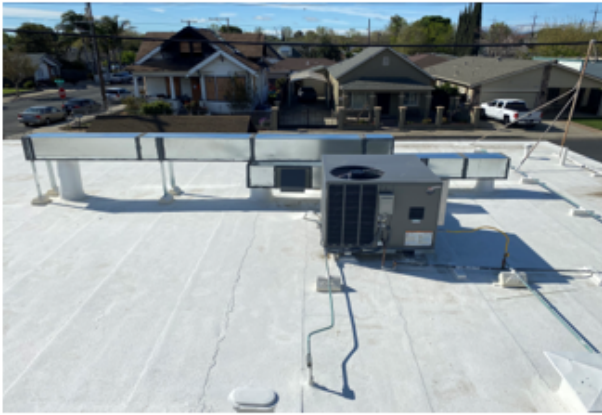
D. Senior Center Roof & HVAC Replacement Project
