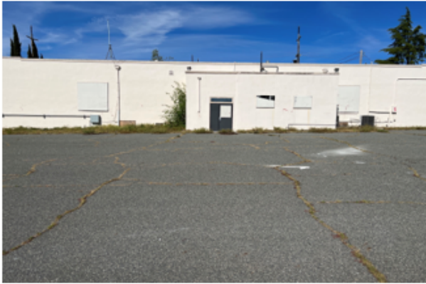
C. Sheriff Annex Building Demolition Project
