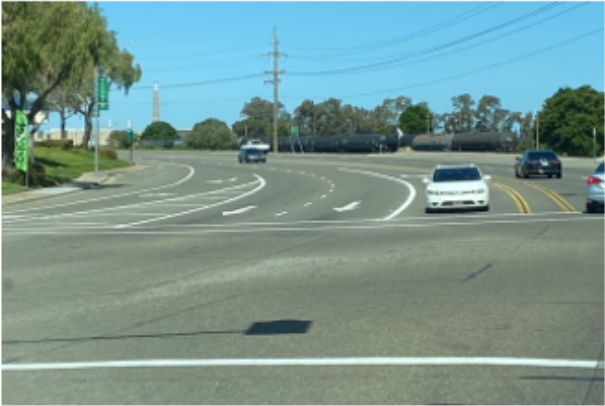
J. Street Restriping Project
