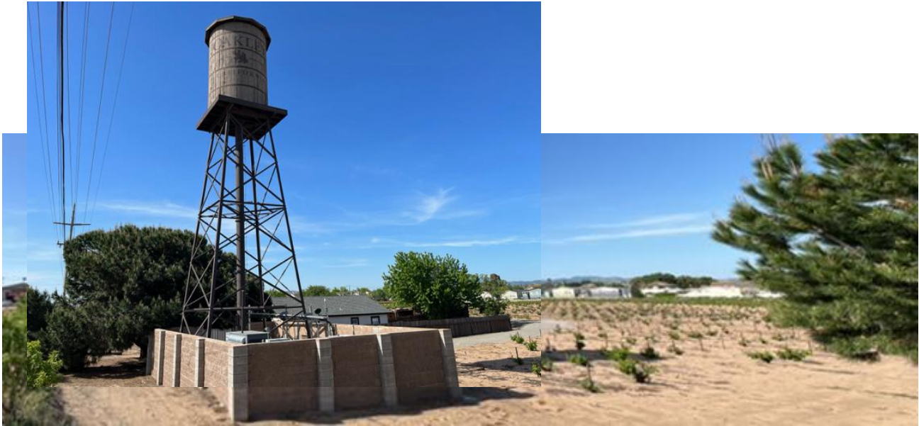
Photo 7: Subject Site (Facing Southwest) Elevator Water Tank and Cell Tower and Associated Vineyard
