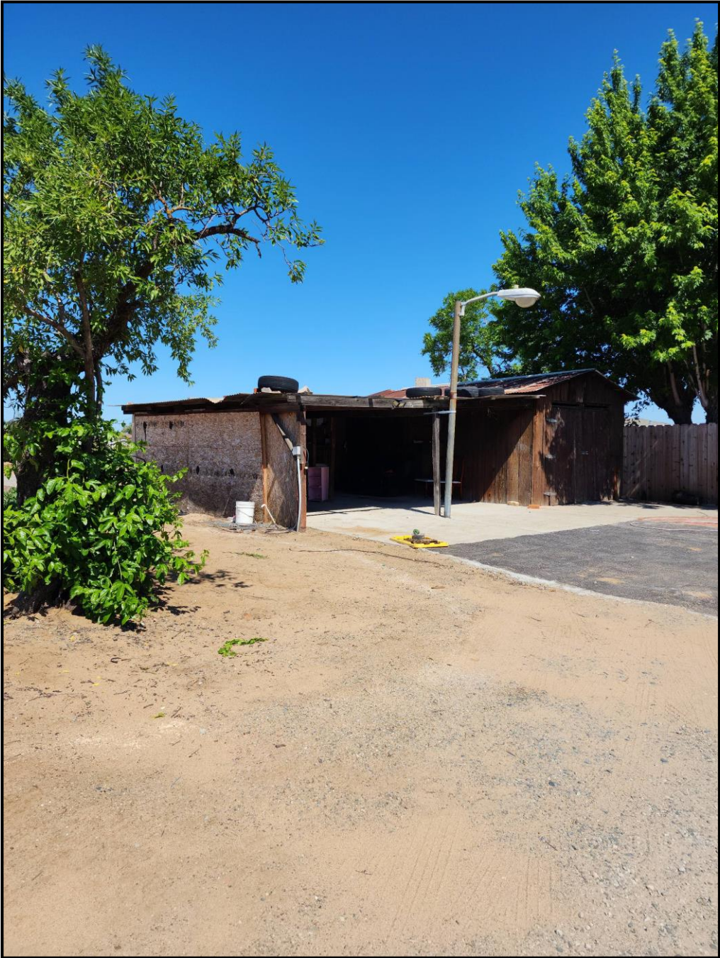
View of shed and carport facing northwest.
