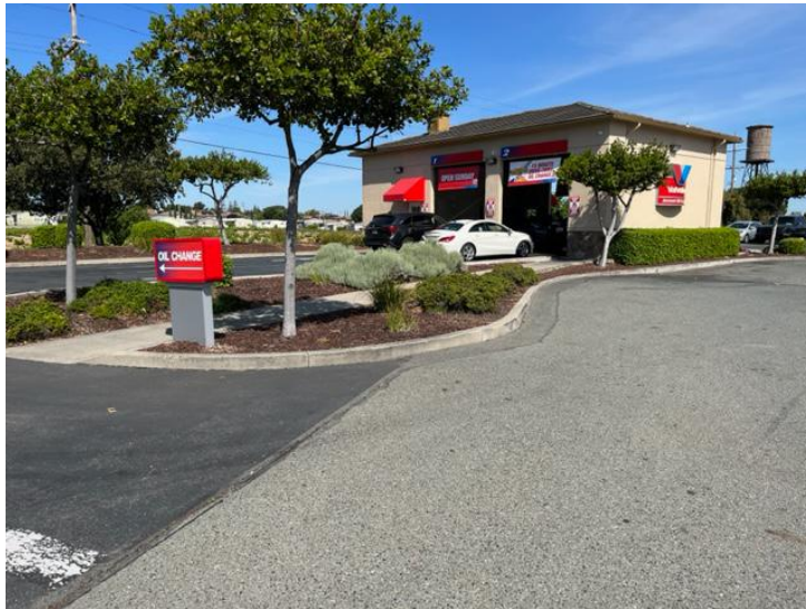
Photo 16: Adjacent Site (Facing Northwest) Valvoline Instant Oil Change Facility (2435 Main Street)
