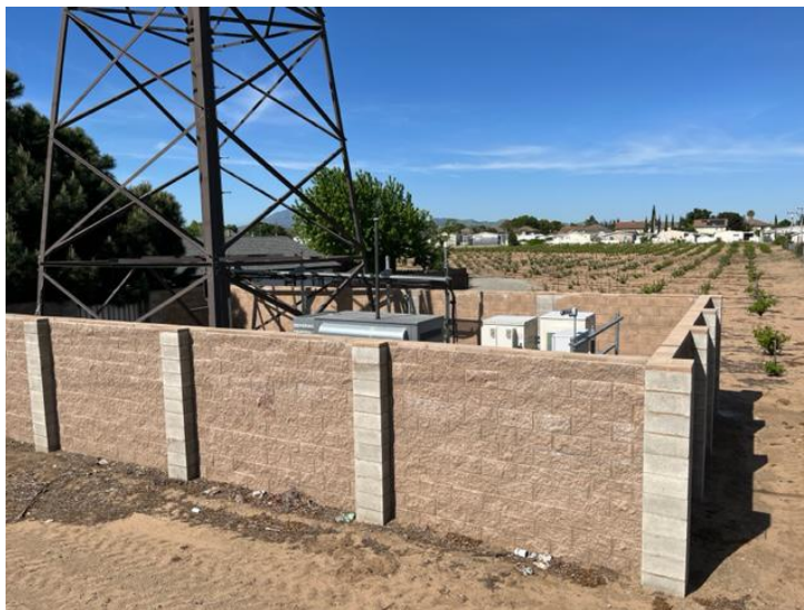
Photo 8: Subject Site (Facing Southwest) Elevator Water Tank and Cell Tower and Associated Vineyard
