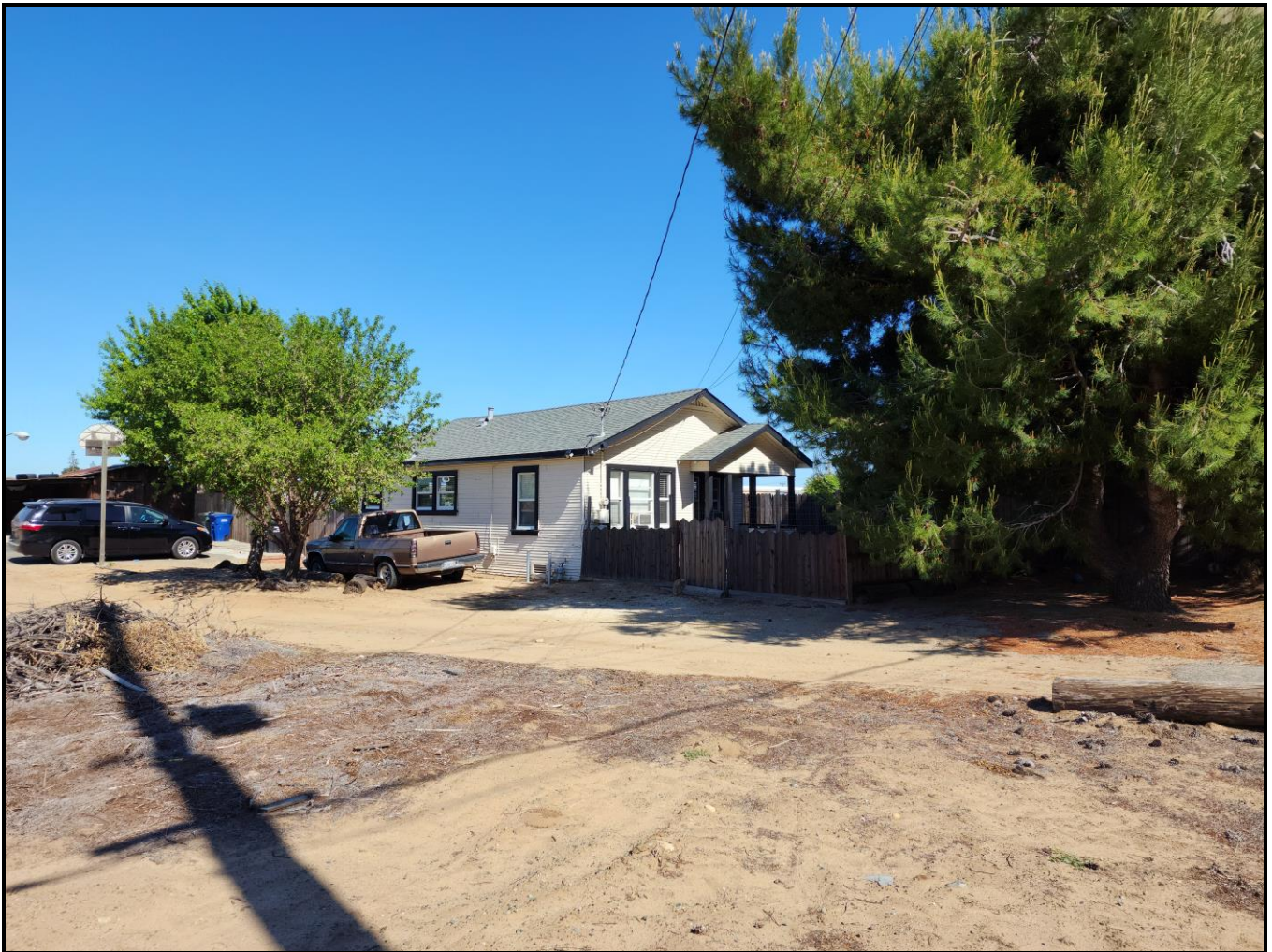
View of house facing northwest.
